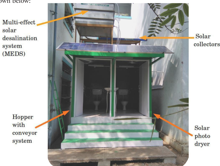
Real time pilot scale zero discharge toilet at IIT Madras
