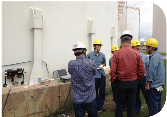
Non-destructive evaluation of the base of an oil tank
